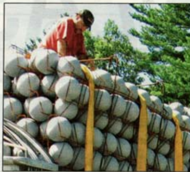
A worker secures blow molded plastic spheres to a truck that will take them to the construction site of Miami's new art museum.
